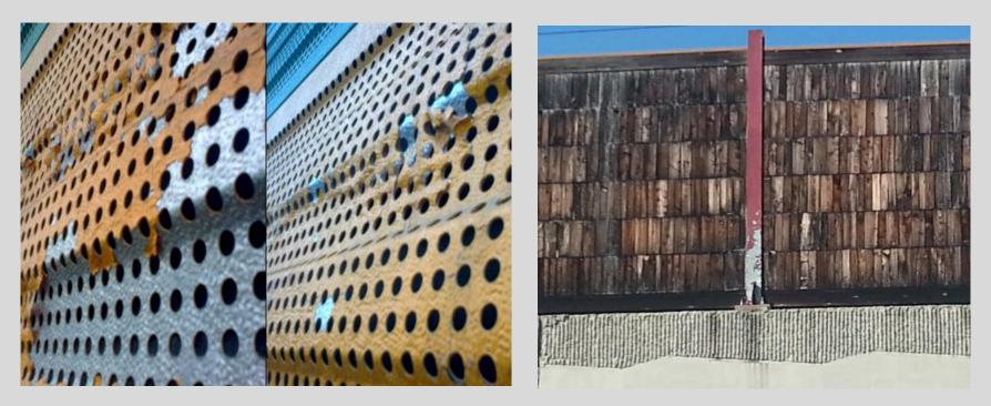
Material specification (corrosion protective layers, wood treatment) are essential for long term durability. Also to be considered assembling system, water drainage..
