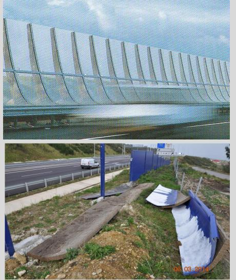
Manufacturers shall declare maximum loads noise barrier are able to withstand provided maximum deflection of post and panels are not exceeded. Loads to be considered are wind load and variable loads due to passing vehicles
