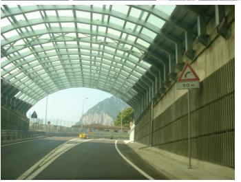
Artificial tunnel built as NRDs for buildings closed to tunnel entrance to save energy used for internal tunnel lighting.
